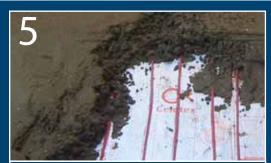
The heating cables are covered with sand and cement screed. Once the screed is dry, the heating should be turned on gradually over a 48 hour period.
