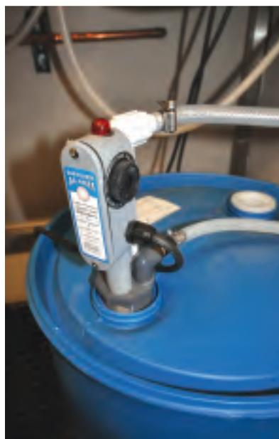
Pick-up tube with low level indicator
