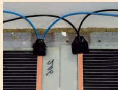
ECOFILM F connection in parallel with Mastic
