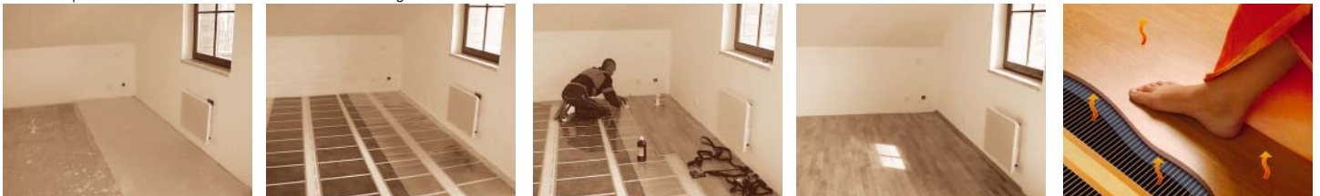
Illustration photo—installation of ECOFILM F608 under floating floor
