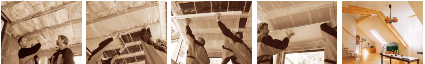
Illustrative photos of ECOFILM C installation on metal joists
