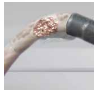
Safety comes first: changing of broken, open insulation
