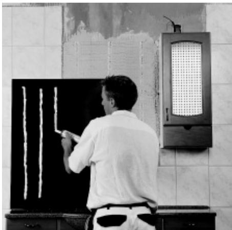
6. The mirror can now be mounted either directly in the tile adhesive or with acid free silicone after the tile adhesive has dried.
