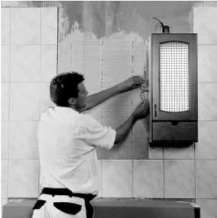
5. Put the cold tails of the heating mat into the flex pipe and push it up to the connection box.
