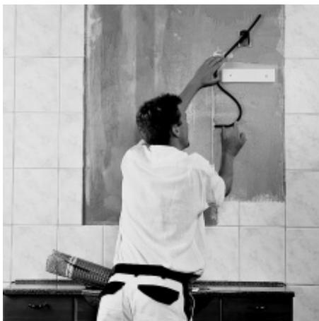
2. Install a flex pipe in the wall from the mirror to the nearest connection box.
