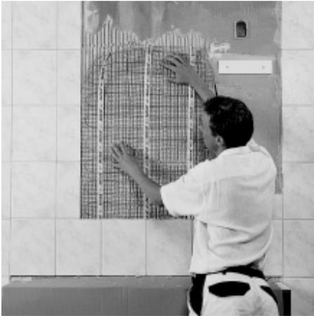
4. Press the mirror heating mat into the tile adhesive - make sure it is even and fixed. Then cover the mat with tile adhesive - make sure the surface is smooth.
