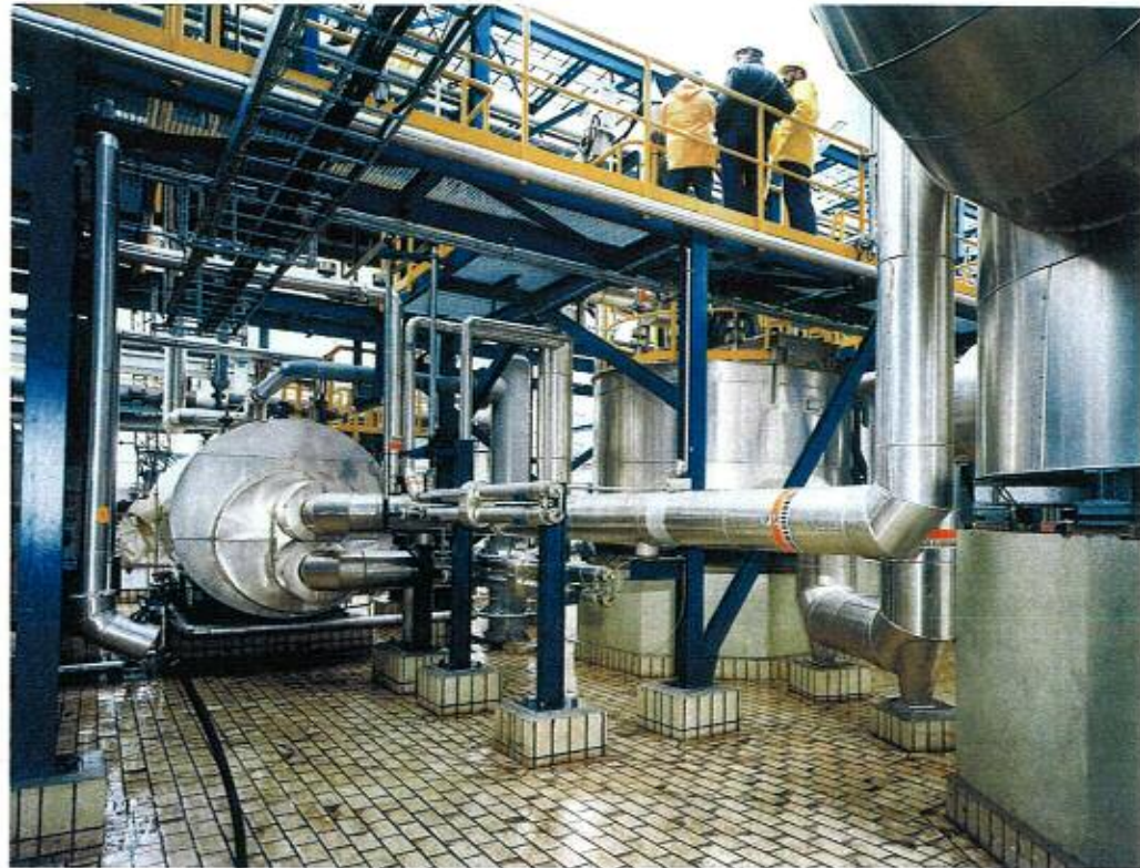
Distributor system of a sulfuric acid plant in Nicrofer 3033-alloy 33. Operator: Norddeutsche Affinerie, Hamburg. Process equipment manufacturer: Franken GmbH, Oberhausen
