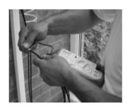
Check the insulation resistance between the conductor and the earth screen, this should read infinity.
