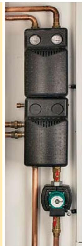
Dual differential pressureless manifold DDV 32
