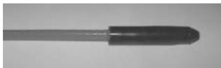
6. The heating cable is sealed / terminated.
