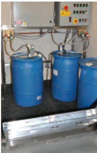
Containment platform with drain pan and leak sensor
