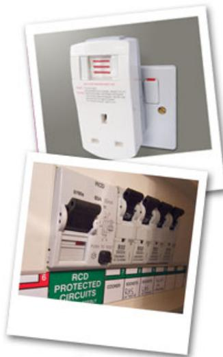
**A residual current device (RCD) is a safety device that switches off electricity automatically if there is a fault.** RCDs are far more sensitive than normal fuses and circuit-breakers and provide additional protection against electric shock.
