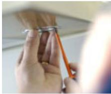
If your wall or ceiling light are not working it will be due to either a bulb that has blown or a problem with the circuit. To find out whether it is just a bulb that has blown check to see if the lights in other rooms are working. If it is a circuit problem then all the lights in one or more rooms will not be working.
