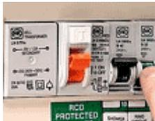
If you are not sure which appliance has caused the problem, unplug all appliances, reset the circuit breaker and/or RCD by switching back on. Plug each appliance back in, one by one, until the faulty item (which trips the circuit) is found.
